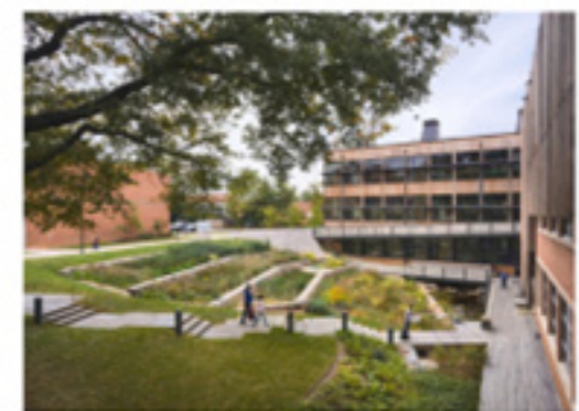
The Sidwell Friends School in Washington, D.C. Depuradora natural
